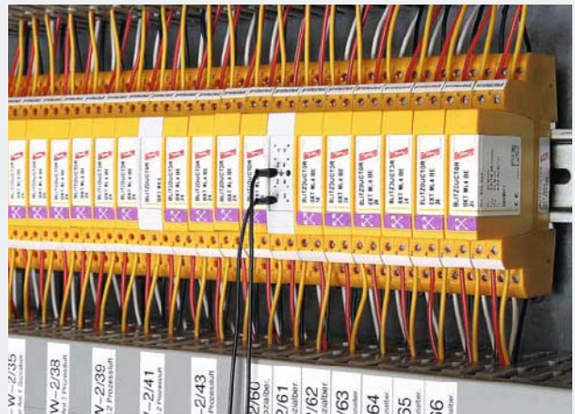
Example of use of BLITZDUCTOR XT with an earthing module (grey). The lines can be tested by means of a measuring module (grey with connecting lines) without disconnecting the terminals.
